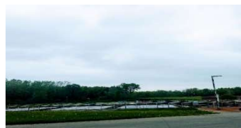
A view of DWTP 2 in Northeast Stark County in Ohio
